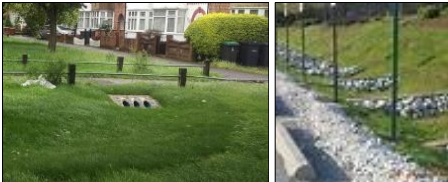
Figure 11 | Examples of Swale Crossings and Check Dams
